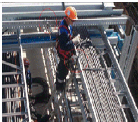
Figure 2: Cable pulling process and posture on tray
